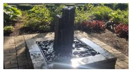
• Workers from Aquascape of were here to rebuild the front garden fountain. The main Basalt columns were stabilized, and new pumping equipment was installed. The fountain was damaged when a small boy and his father accidentally knocked down the 3 Basalt columns, damaging the equipment below. As you can see the result was quite good, better than the original in fact.
